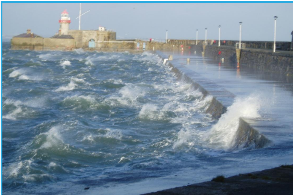
Figure 4 Overtopping in Dun Laoghaire Harbour
